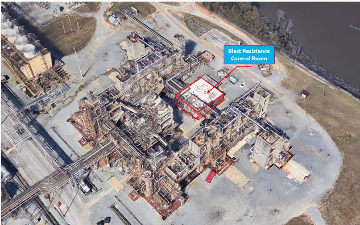
Figure 6: Control Room Revalidation
