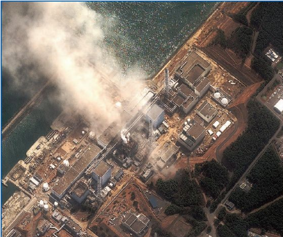
Earthquake and tsunami damage at the Fukushima nuclear power plant
